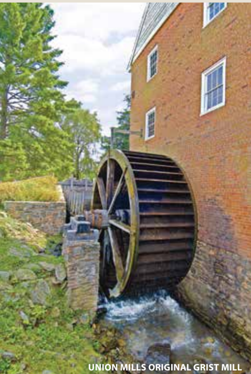
UNION MILLS ORIGINAL GRIST MILL
